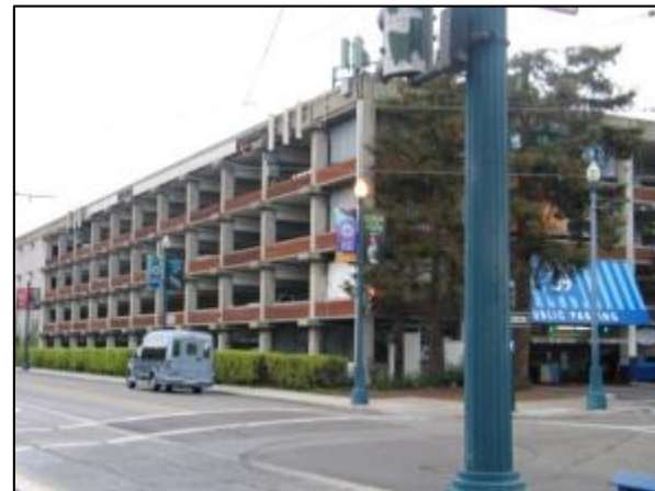
Photograph 4. Stockton Street facing east toward the Pier 39 parking structure.
