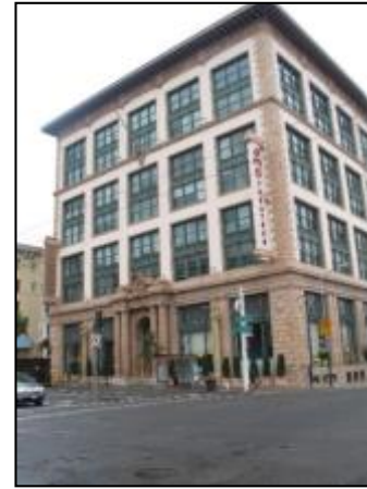
Photograph 52. Dan Lee Automobile Showroom Building at 1000 Van Ness Avenue, to the north of ES-10.
