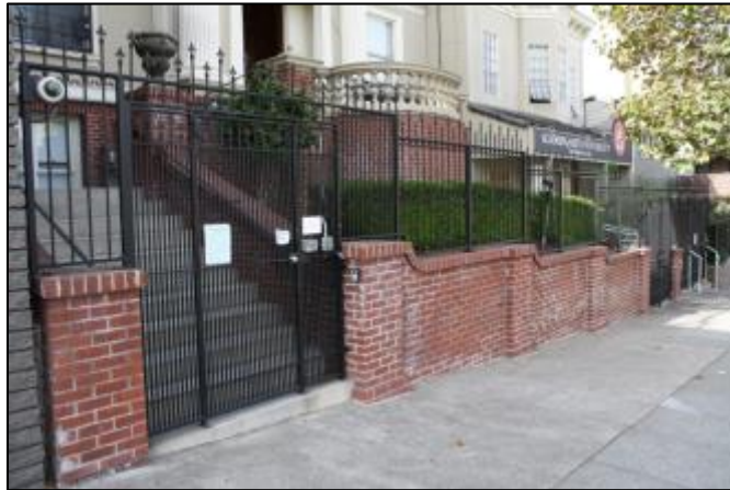
Photograph 31. 2209 Van Ness Avenue, close up of the yard and security fence on the primary elevation
