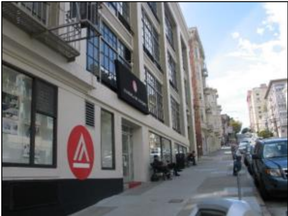
Photograph 40. Mid-block Washington Street, facing west.
