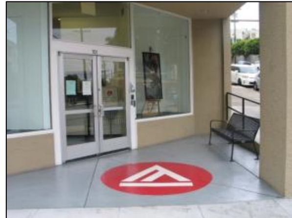
Photograph 11. Main entryway to ES-2.
