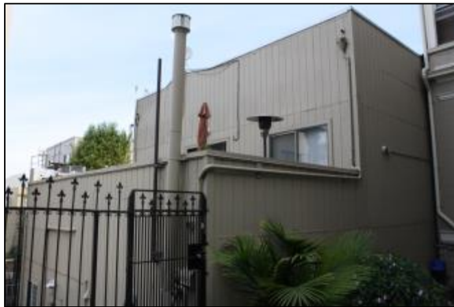
Photograph 26. 2211 Van Ness Avenue, northeastern perspective of the upper stories of the west elevation
